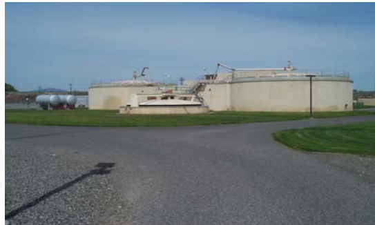
Anaerobic Digesters
