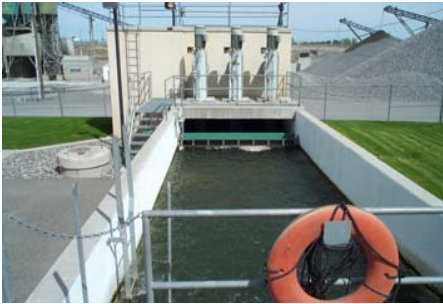
Chlorine Contact Chamber
