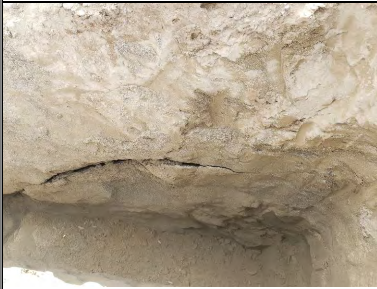
Exposed subsurface soil profile to ~9' BGS within test pit P-1
