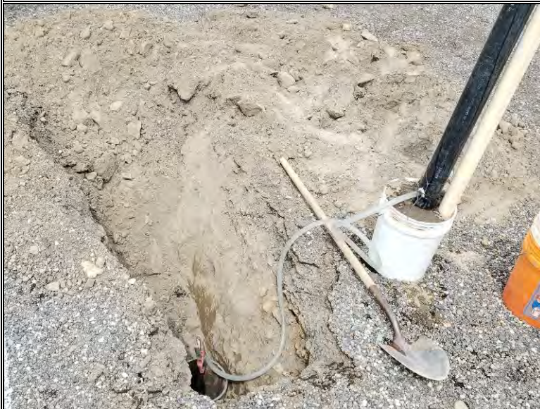
Infiltration test setup at test pit P-2
