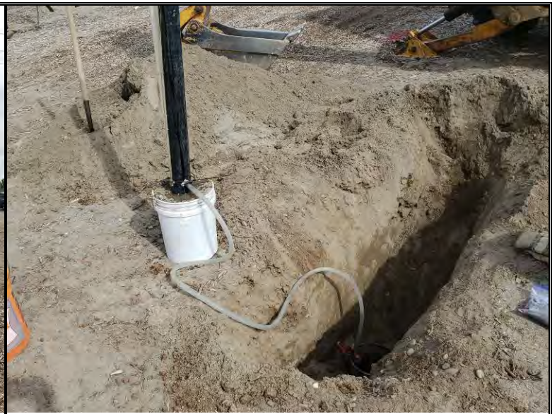
Infiltration test setup at test pit P-1
