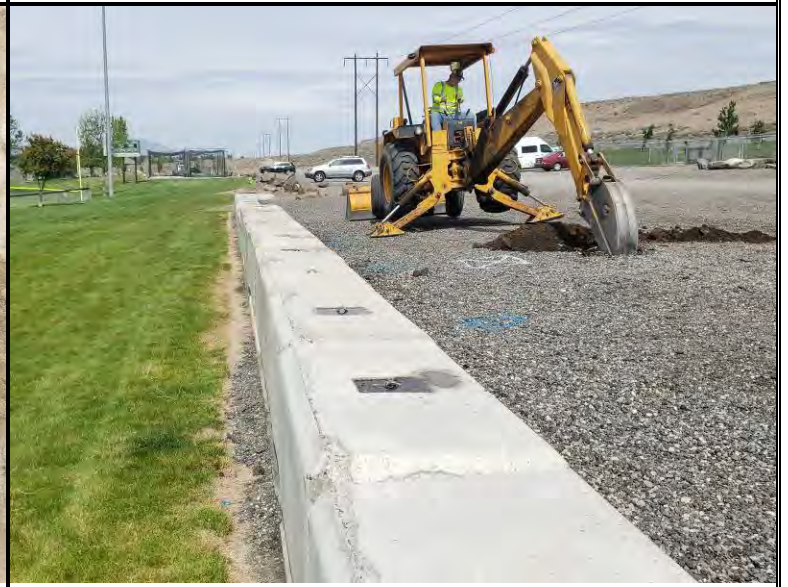
Excavation of test-pit P-2, looking west
