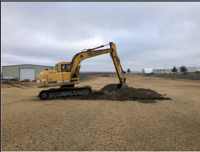
Excavation at test-pit TP-3, view looking east
