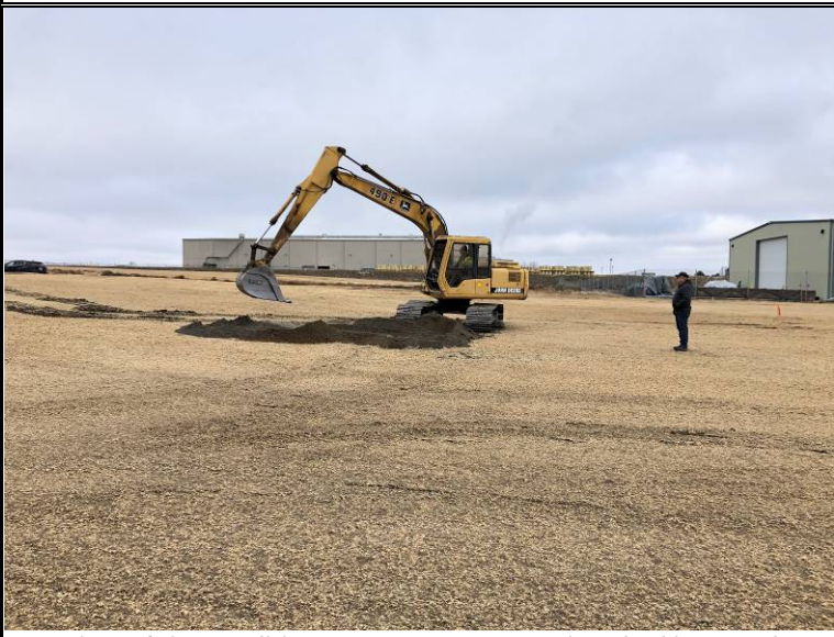
View of site conditions across eastern portion, looking north
