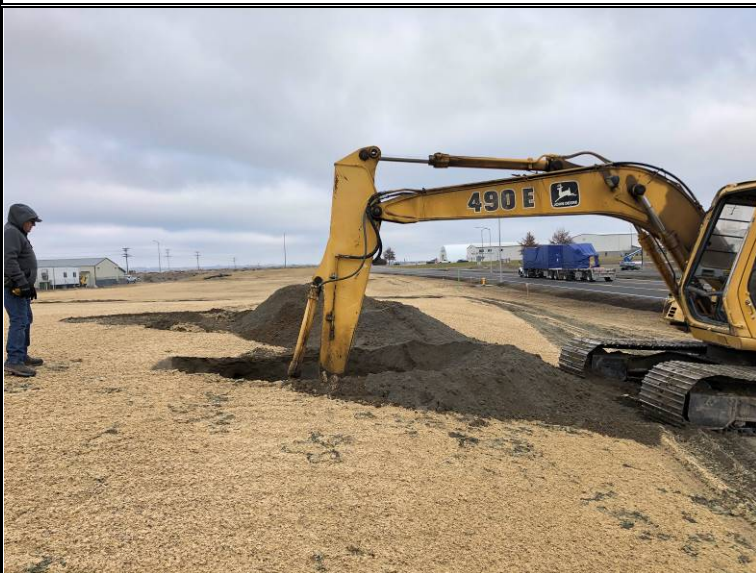
Excavation at test-pit TP-6, view looking east
