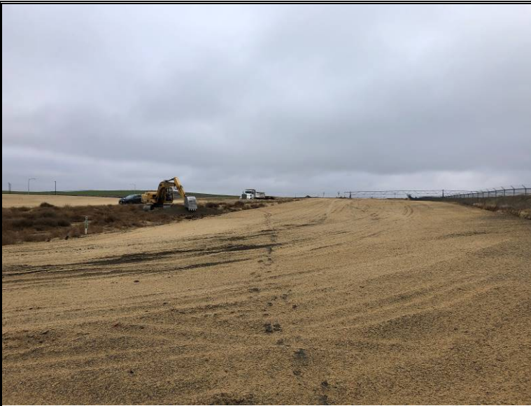
View of site conditions across northern portion, looking west
