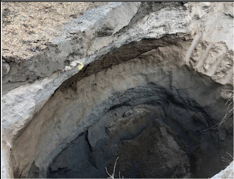
Exposed soil profile within test-pit TP-1
