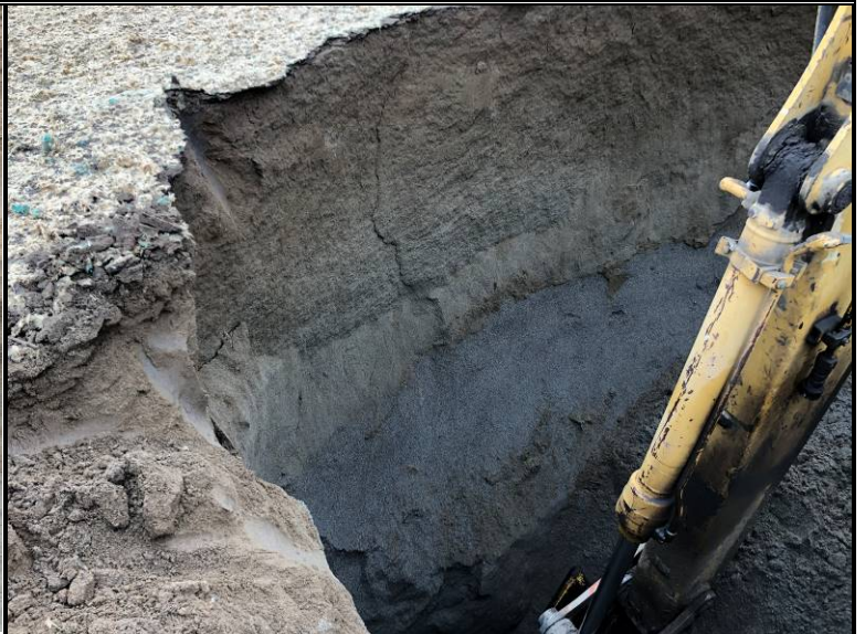
Exposed soil profile within test-pit TP-5
