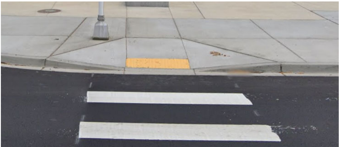
Figure 2-2 - Example of Perpendicular Ramp
