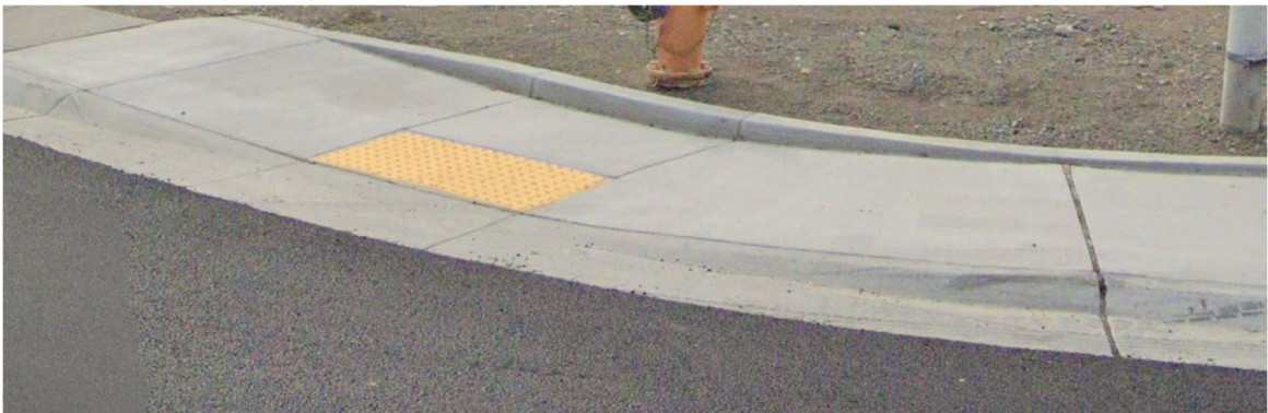
Figure 2-3 - Example of Parallel Ramp
