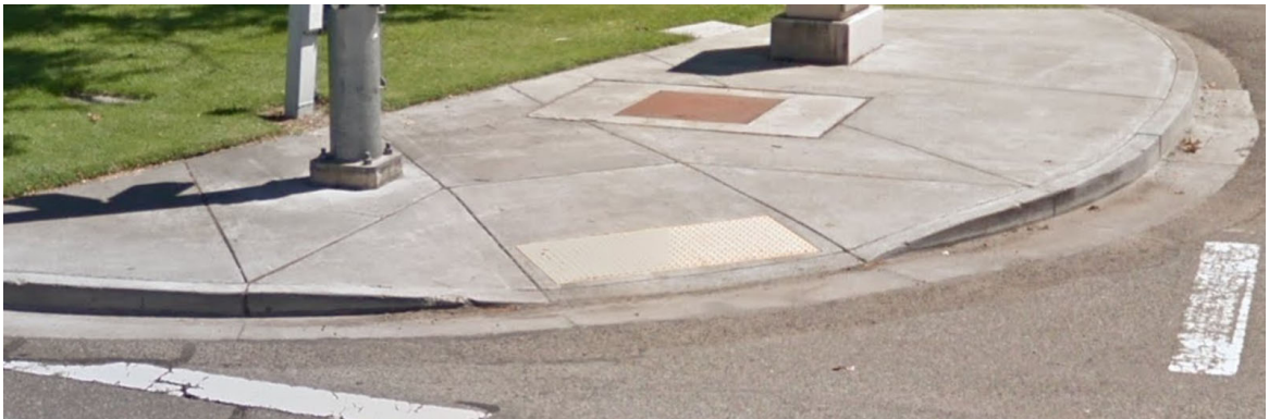
Figure 2- 4 - Example of Diagonal Ramp
