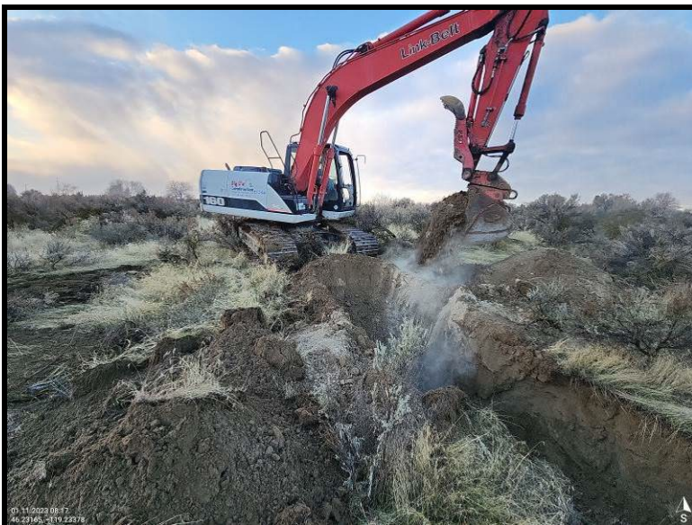
Excavation of test-pit TP-1
