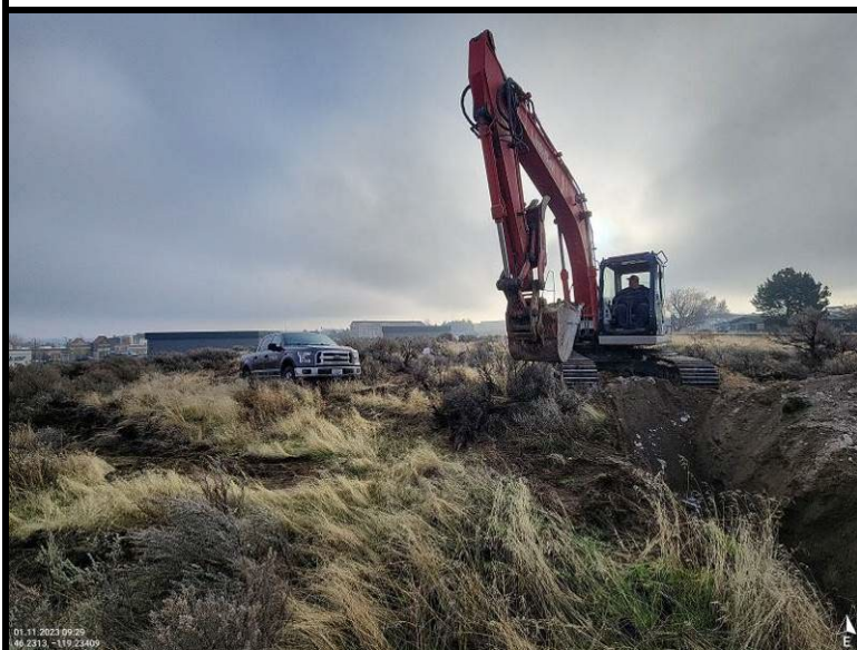
View of site conditions looking east from test-pit TP-4
