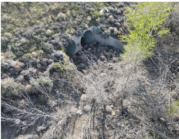
Photo 7. East Badger Drain culvert under I-84
