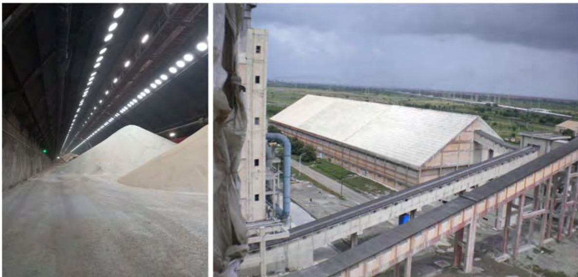
Figure.6. Example of shelter for CAN storage indoor/outdoor.
