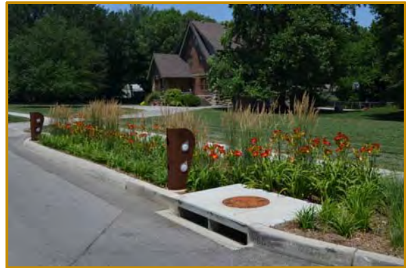
Example photo of a preferred curb inlet with sump into a bioretention facility (likely oversized).
