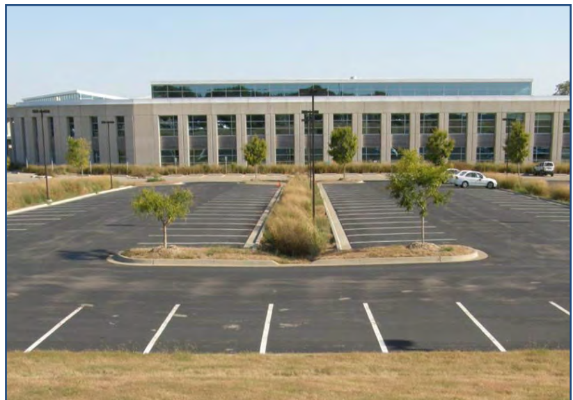
Example non-xeriscaped parking lot bioretention swale.
