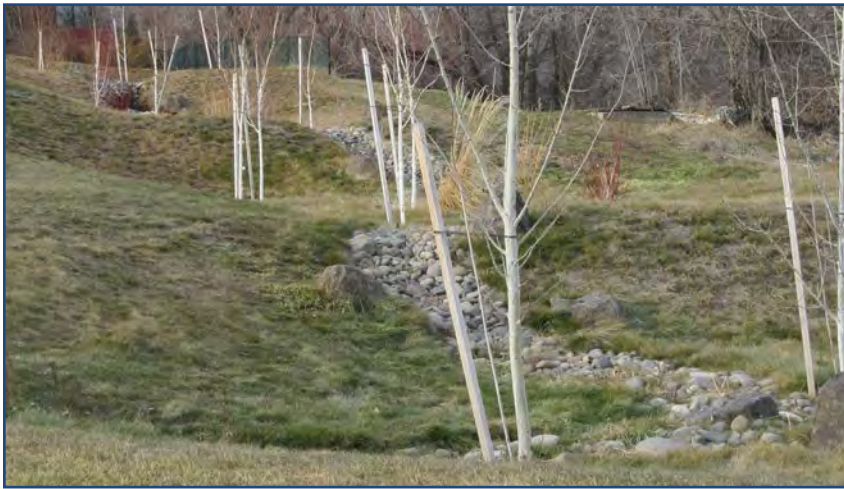
Example of cascading bioretention swales.
