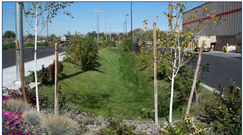
Example bioretention swale. Lower zone comprised of turf grass and upper zone comprised of select grasses, shrubs, and trees.
