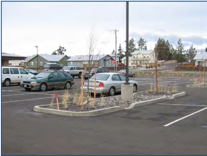
Example xeriscaped parking lot bioretention swales.
