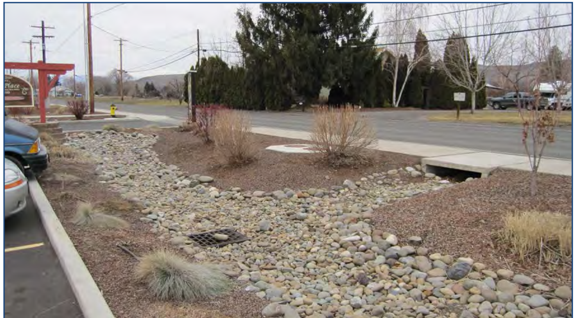
Example bioretention swale with a xeriscaped approach. Lower zone comprised of river rock and upper zone comprised of select grasses, shrubs, and trees.
