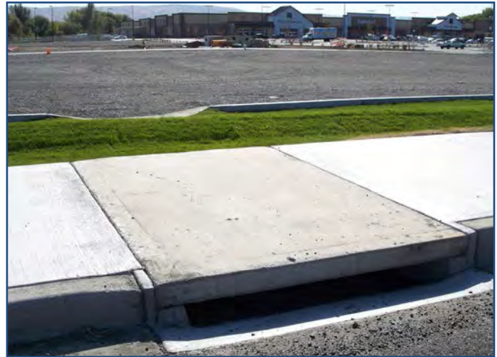
Example bioretention swale with roadside and parking lot runoff inputs. Note the berm separating the roadside swale from the parking lot swale.
