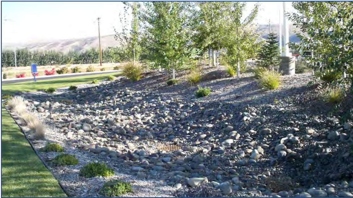
Example bioretention swale with a xeriscaped approach. Lower zone comprised of river rock and upper zone comprised of select grasses, shrubs, and trees.
