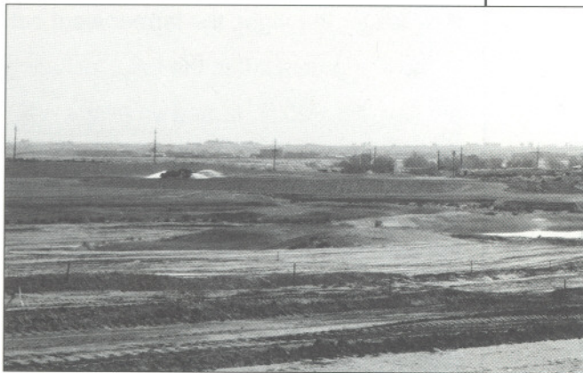
Preliminary golf course construction for the planned community at Horn Rapids, 1993.
